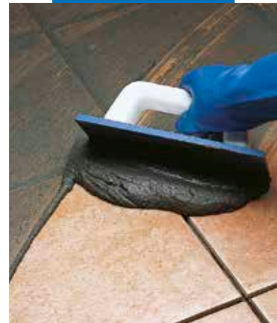
Grouting single-fired tiles with a float
