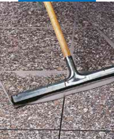
Grouting of pre-smoothed and glossed granite floor with rubber float
